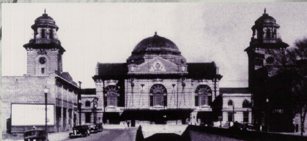
Birmingham Terminal Station
